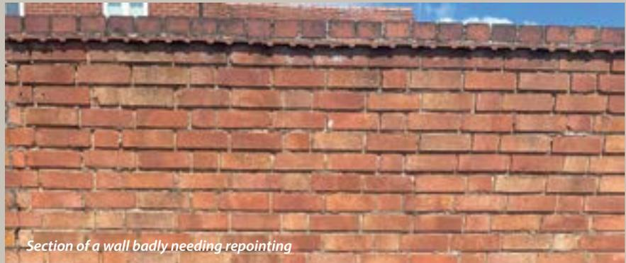
A data sheet, 'Repointing external brickwork', explains that mortar in poor condition can lead to a loss in wall strength. This is often found in old properties where mortar is powdery or easily scraped away so that the joints are appreciably recessed. Incorrect use of pressure cleaning of fresh mortar in new masonry can also affect the strength of new construction and must be avoided.
