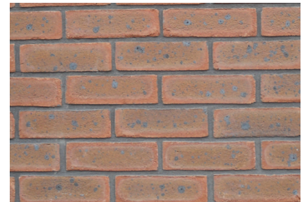
Detail of the b2net stadium's brickwork
