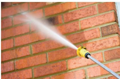
However, if there is extensive splashing, careful washing using a diluted acid solution and low pressure water may be required but this should only be carried out when the mortar is deemed to have cured, probably at least after more than 28 days after application, the generally accepted minimum curing time for cement-based products.
