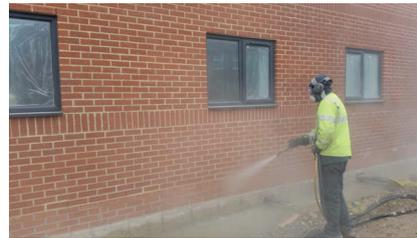
Mortar splashes may be treated with a dilute hydrochloric acid solution, as bricks and joints should be assumed to be moderately to highly porous to chemical cleaner. Concentrated hydrofluoric acid-based cleaners should not be used and any acid solution should be washed off with clean water as quickly as possible. However, rinsing water should not be applied at excessively high pressures, or through an unsuitable nozzle. This is explained further in below.
