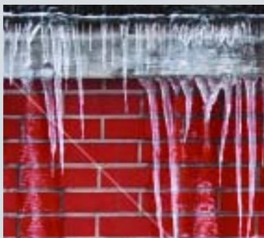
If the temperature of recently laid mortar falls below 0°C there is a probability of some degree of frost attack. The water may freeze and expand thus disrupting the mortar by forcing the material apart and breaking the bond.
