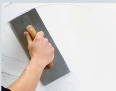
The use of lime and cement in plastering mixes, provides highly workable mortars which are easy to apply - durable - quick to dry out - and minimise the risk of efflorescence, condensation and pattern staining. In damp conditions where other plastering systems may fail, cement:sand and cement:lime:sand plasters are satisfactory. Finish coat plaster is generally gypsum-based and is outside the scope of this data sheet.
