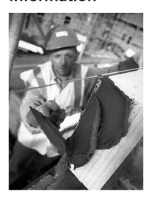
Factory produced ready-to-use mortars fulfil the requirements of specifiers and users seeking factory made materials. They are delivered to site ready-to-use in every respect and require no further mixing; no further constituents should be added. They have guaranteed mix proportions and overcome any potential problems relating to site mixing.
