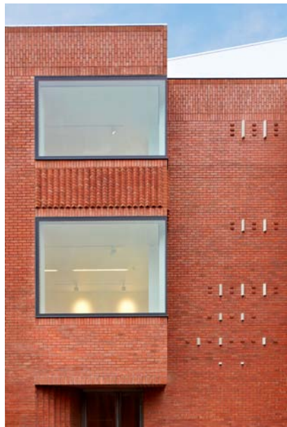
Internal and external brickwork at the Whitworth Art Gallery
