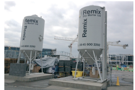
Silos on site at Heathrow ensure readily available mortar supplies
