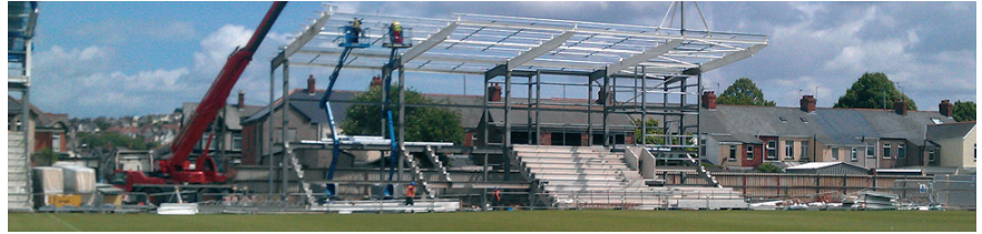
The new stand under construction
