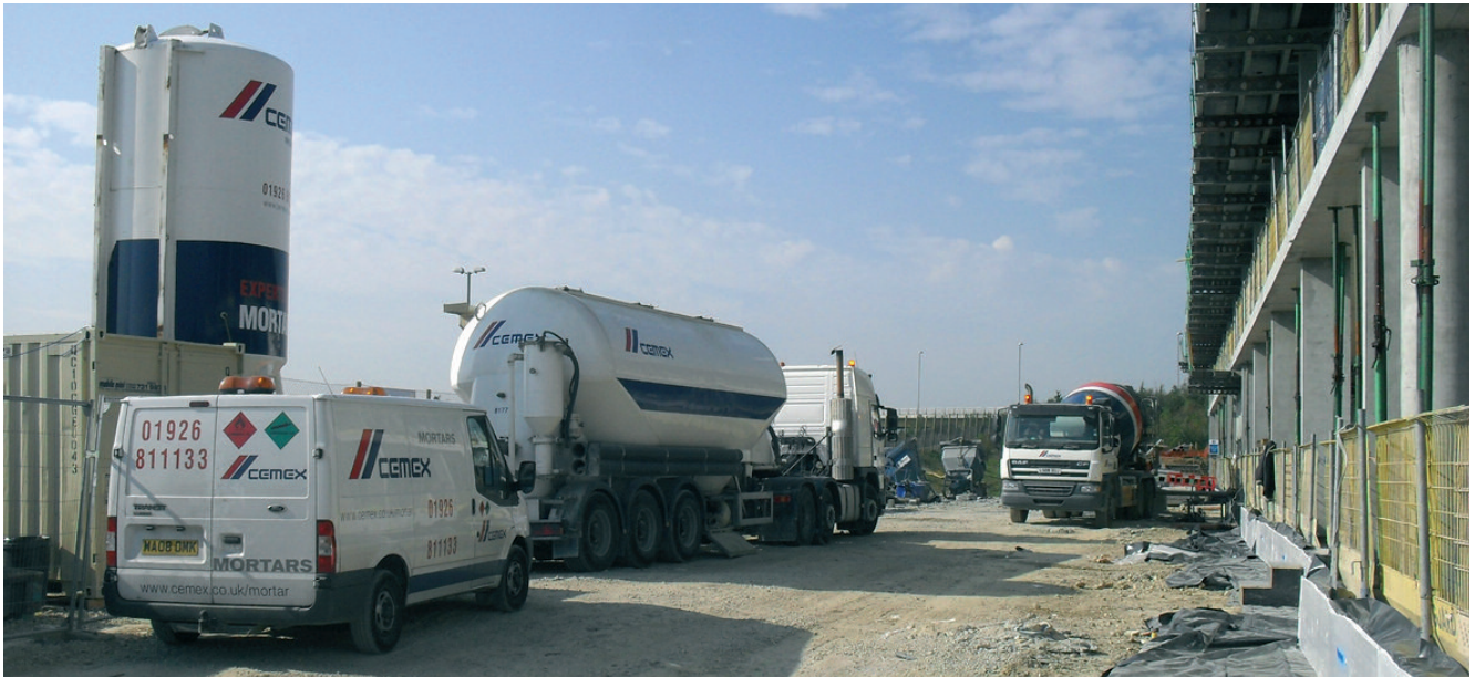
Site for the new Premier Inn by Stansted Airport
