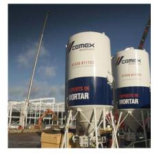
used silo sizes are from 18 to 22m<sup>3</sup>, which hold between 27 and 35 tonnes. Various smaller sizes are also available, which are available in sizes as small as 6m<sup>3</sup>, with a capacity of 9 tonnes. These smaller silos may be delivered by crane offload vehicle, with two per vehicle allowing a delivery vehicle to visit two sites.
